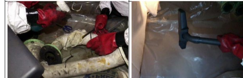
Vacuuming done across the area after the work is completed
