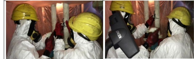
Removal of ACM with spraying of water
